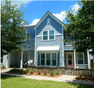
Figure 5.12 The first photo above shows a building frontage dominated by a garage and drives, creating an auto-centric environment. Contrastingly, the photo below includes a frontage type, which creates a more pedestrian-friendly experience.
