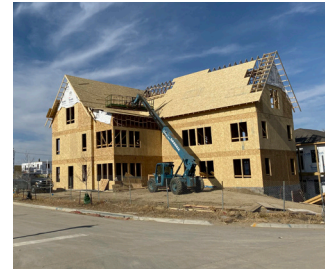
Figure 2.5 The simple forms, smaller size, and compatibility with Type V construction help maximize affordability and investment returns, and are consistent with the construction strategies familiar to most residential homebuilders, as shown in this under-construction MMH project in Papillion, Nebraska.
