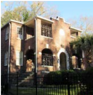
Figure 2.12 Example of projecting porch MMH frontage in Columbia. Upper-story units in the building are accessed by a single, shared entry that leads to a hall or small lobby area.
